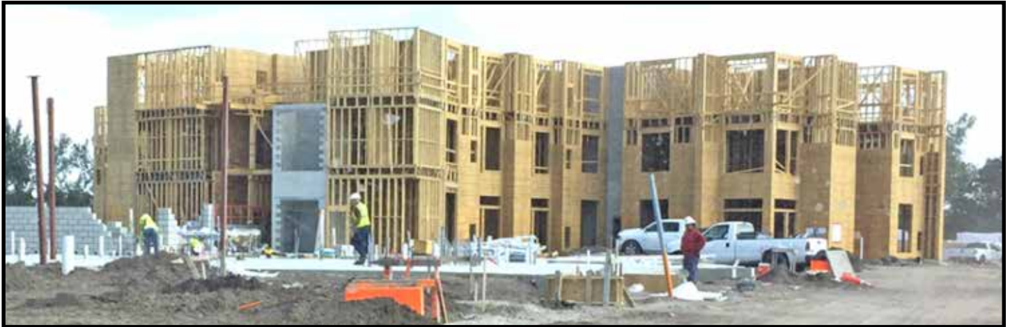
Construction progress as of September 30, 2019 ~ Photo by Pam Babbitt
