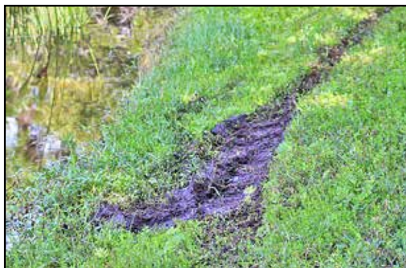
Egret Pond bank failure and shoreline damage by mowing too close to shore, July 2018.
